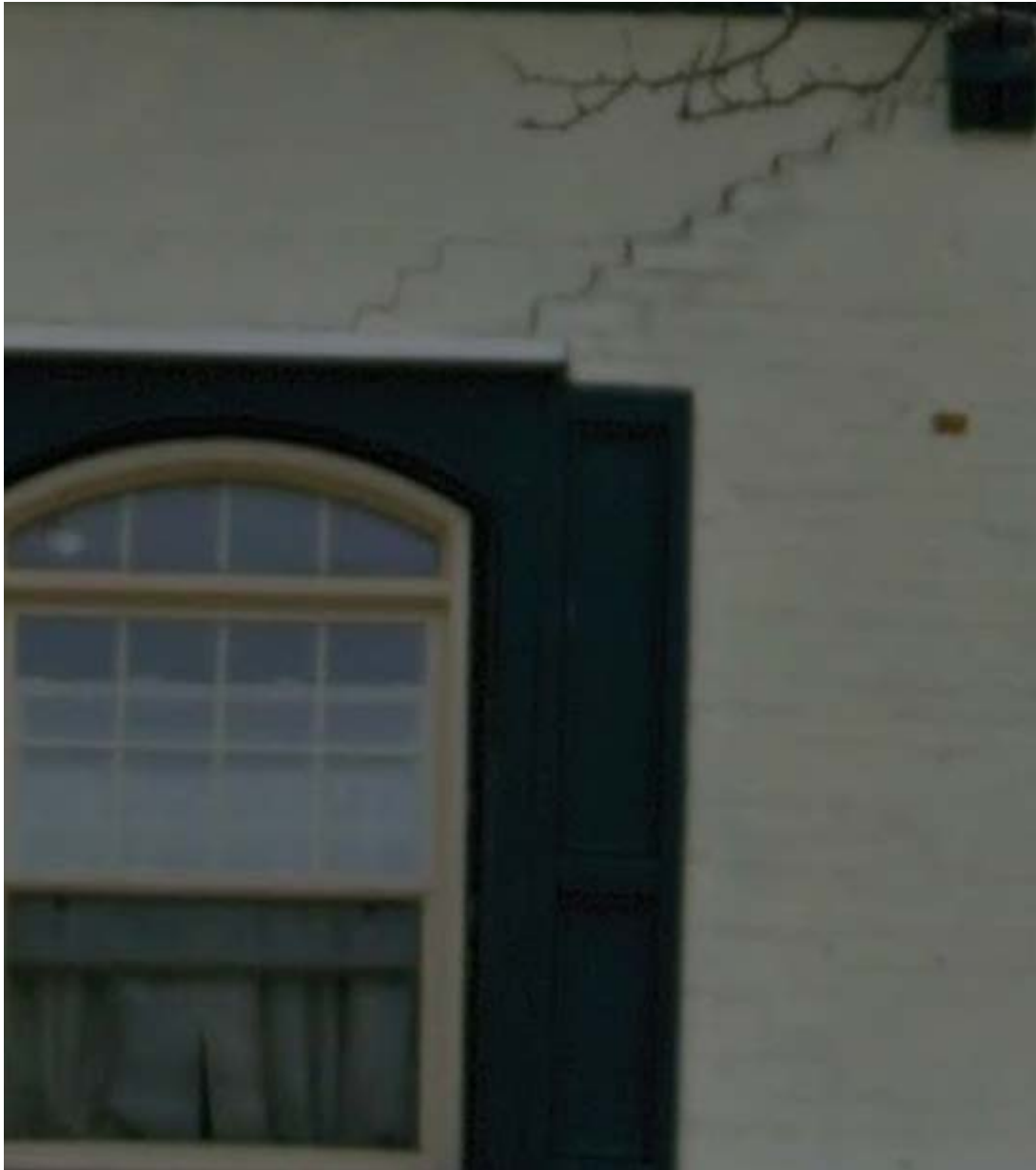
Figure 7: 264 Division St. Masonry crack to be repaired.
