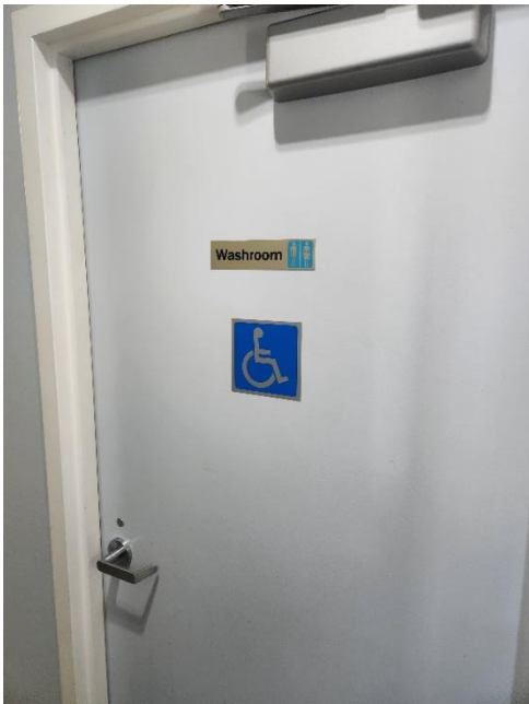
Photograph # 3 Public Washroom with Door Opener
