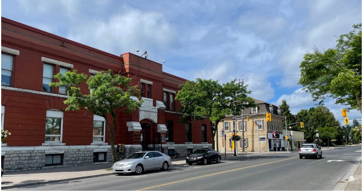
Fig. 4.1.1.1 – Existing Building at 107 King Street West
