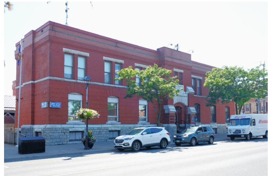
40. The building as seen from the NE. PGA
