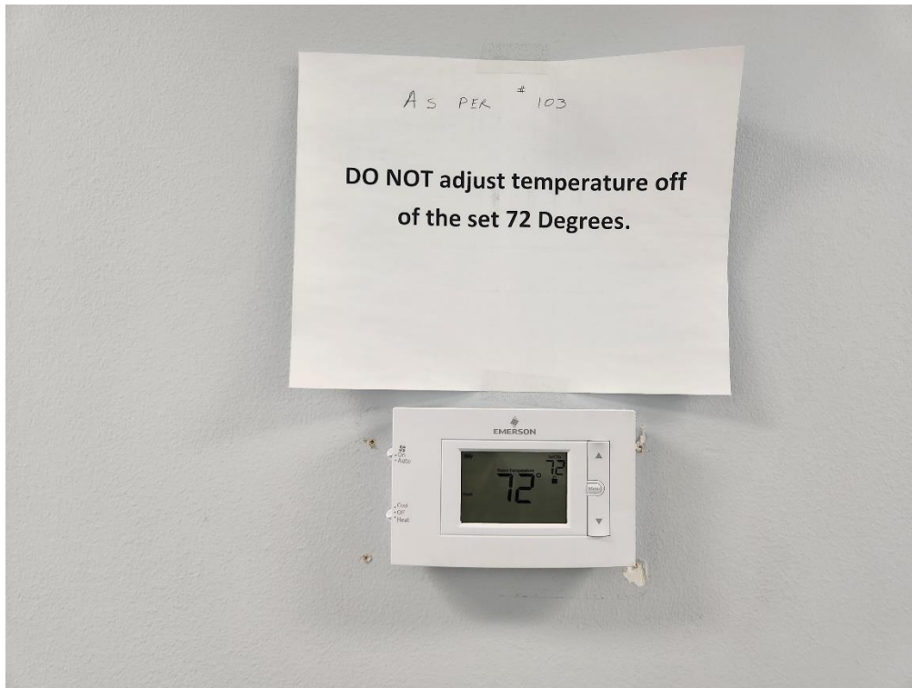
Photograph # 14 Rooftop Unit Controller
