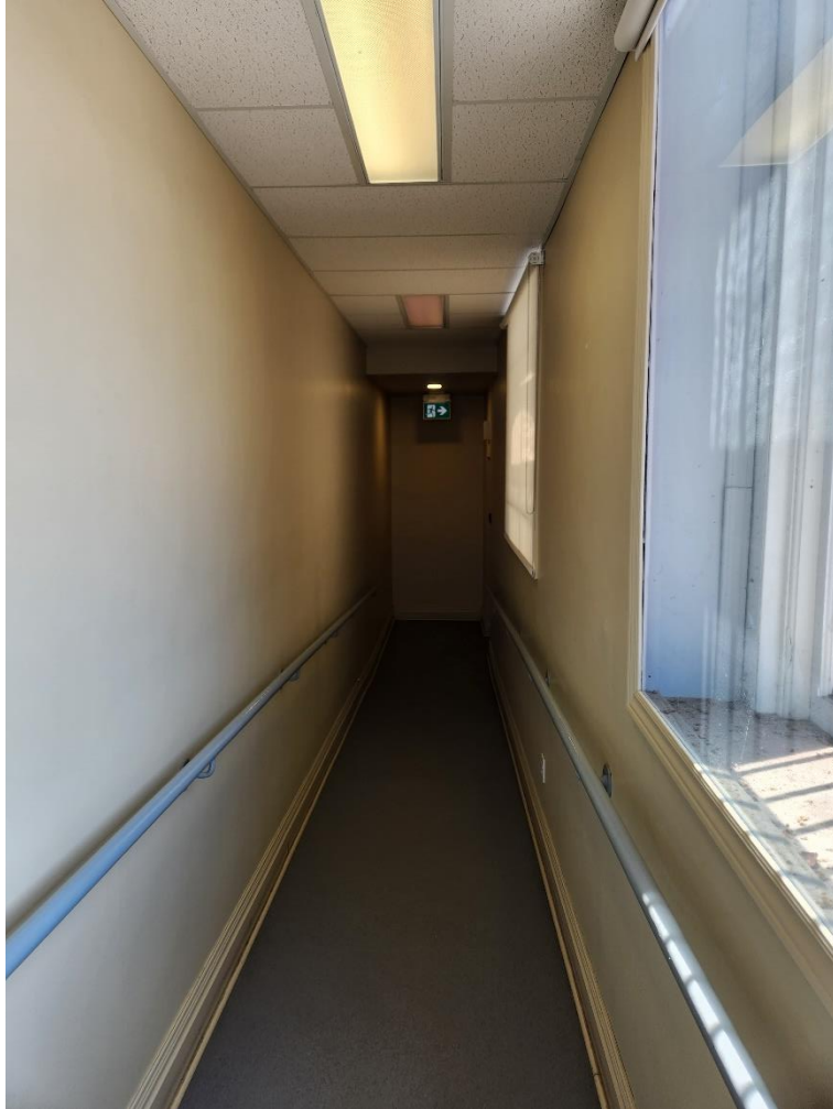
Photograph # 74 1 by 4 Ceiling Mounted Lights
