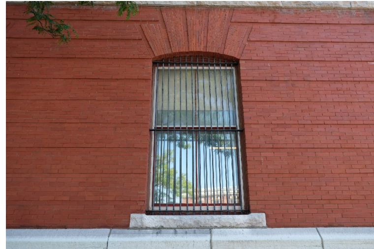
59. Detail of typical first floor 1/1 wood window with protective metal bars. PGA
