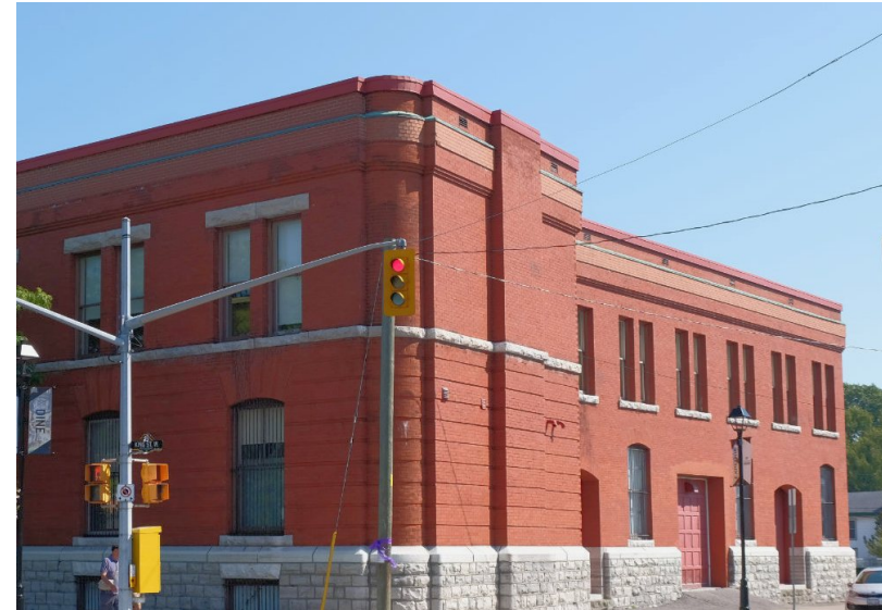
70. The NW corner today, note changes to the parapet-cornice. PGA
