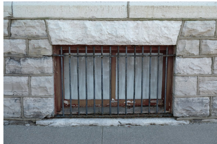
61. Detail of typical basement window . PGA
