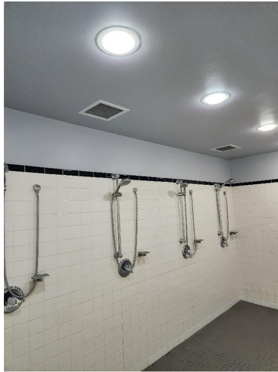
Photograph # 9 Men's Changeroom Showers
