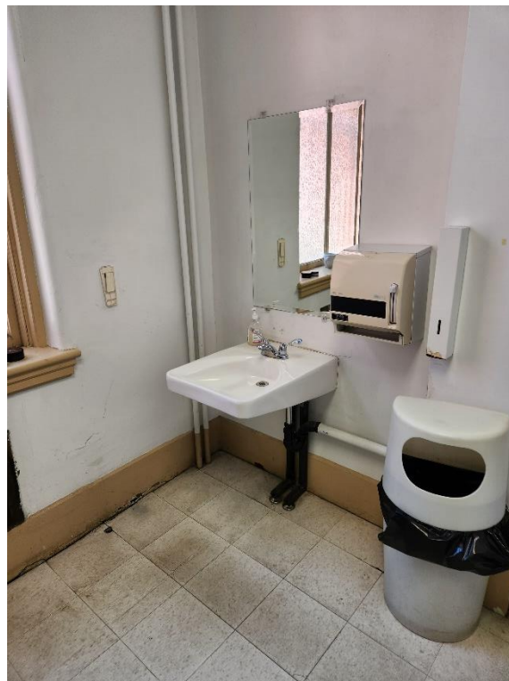
Photograph # 15 Public Washroom Space
