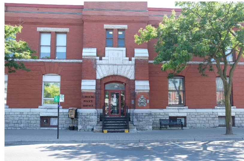
53. Central bay of the north elevation, note changes at the parapet level all around the building compared to the image above. PGA
