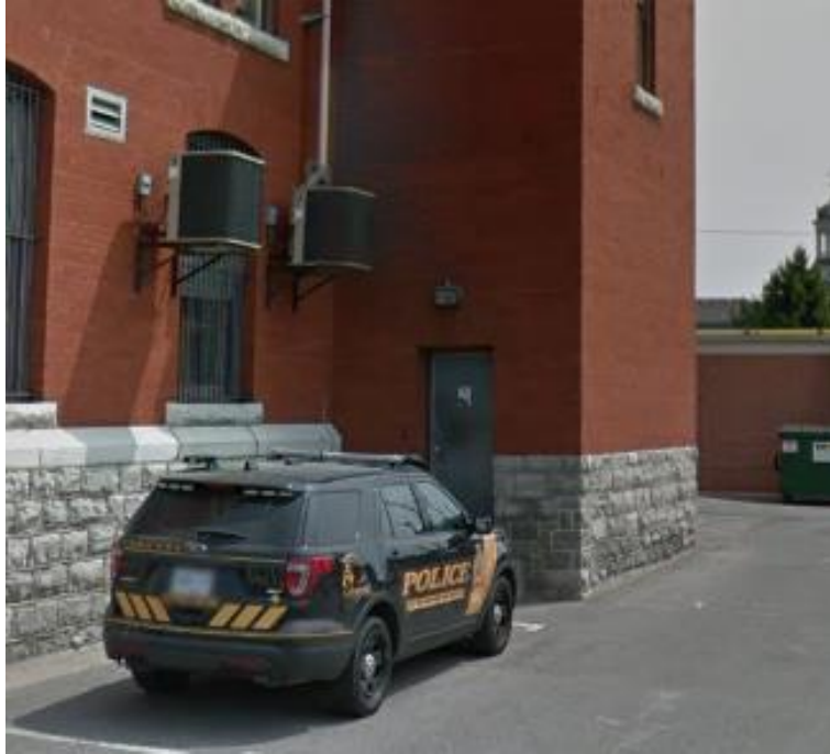
Photograph # 36 Outdoor Condenser Units Connected to Olsen Furnaces
