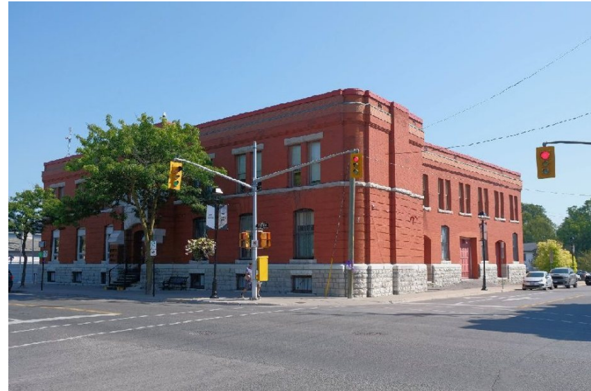
41. The building as seen from the north-west. PGA
