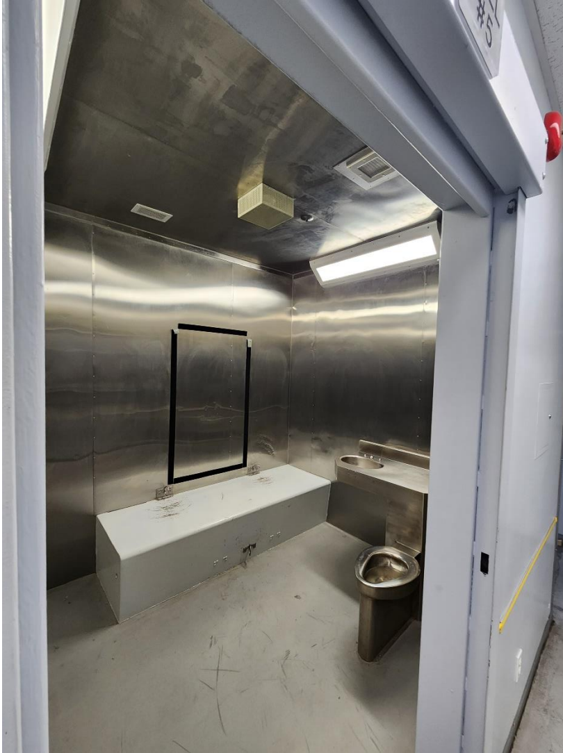
Photograph # 2 Holding Cell Amenities
