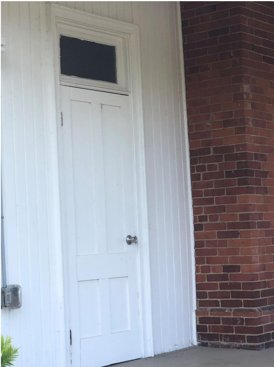
Figure 4: 586 Osler Court mudroom entrance
