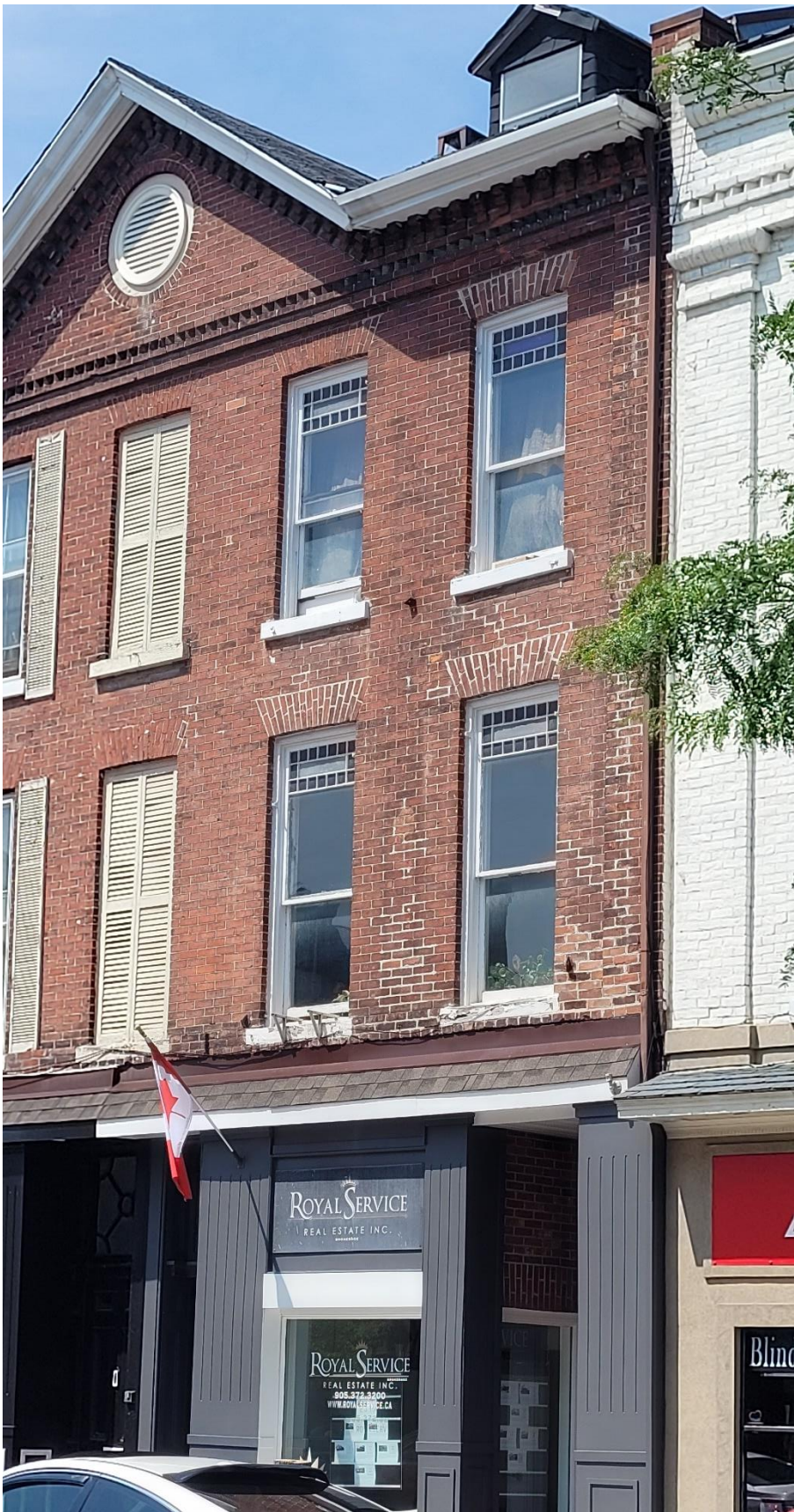
Figure 2: 36 King St. W – Storefront
