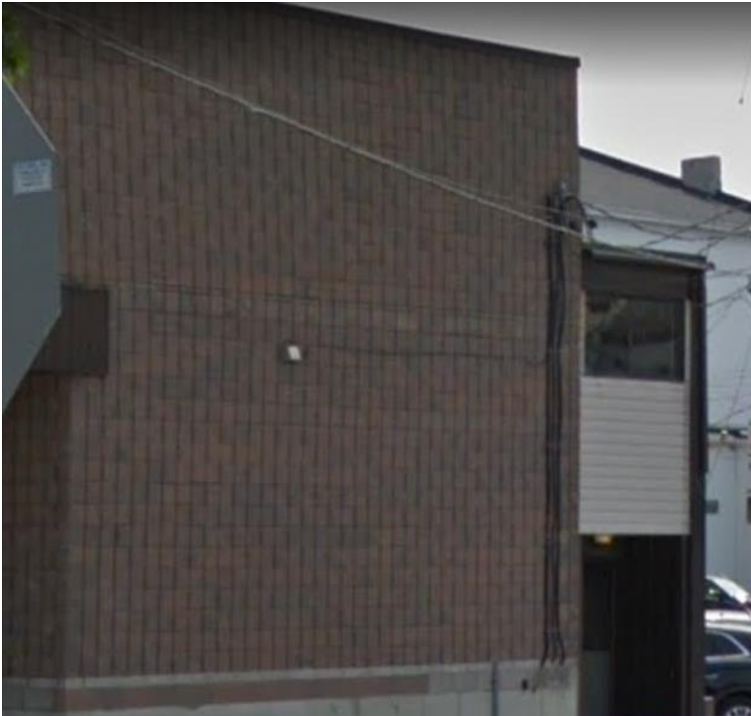
Figure 2: 259 Division west elevation – residential structure showing existing conditions. Image courtesy: Google
