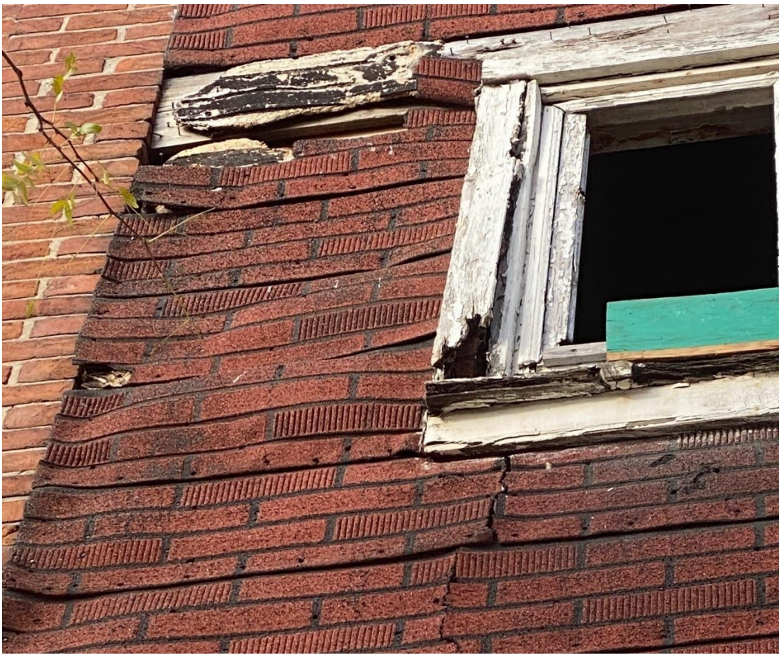
Figure 6: Subject property at 18 King St. E – showing third floor façade damage.
