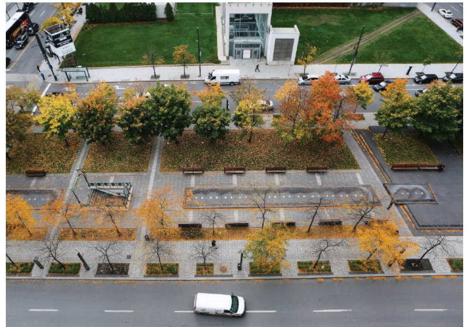
Permeable pavers and gardens increase infiltration
