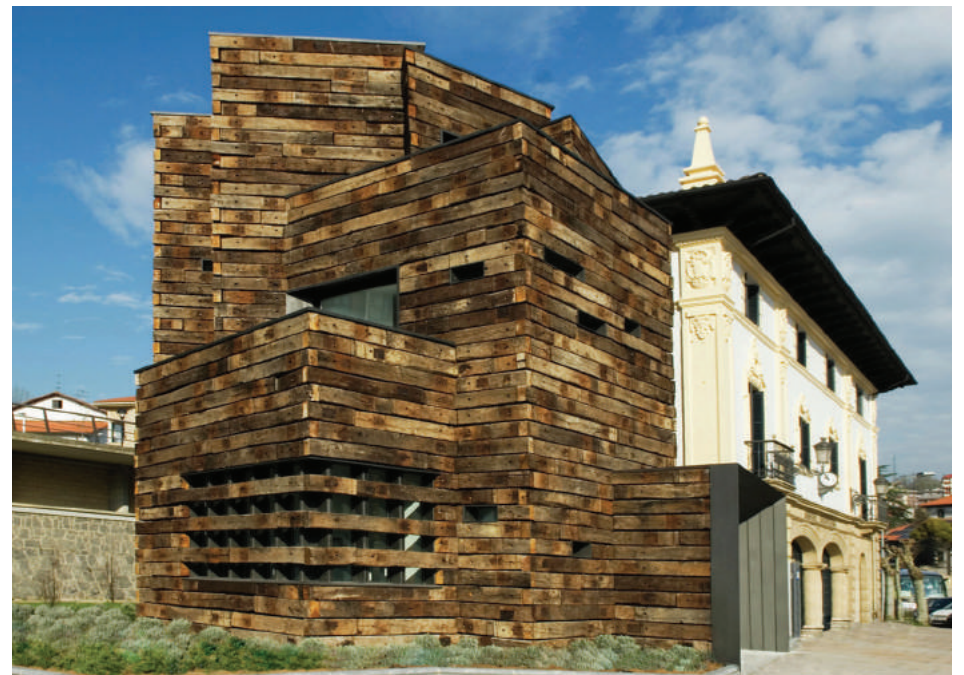
Innovative use of local materials (railroad ties)
