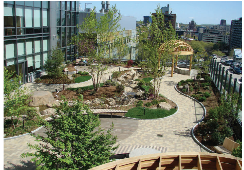
Active Green Roof
