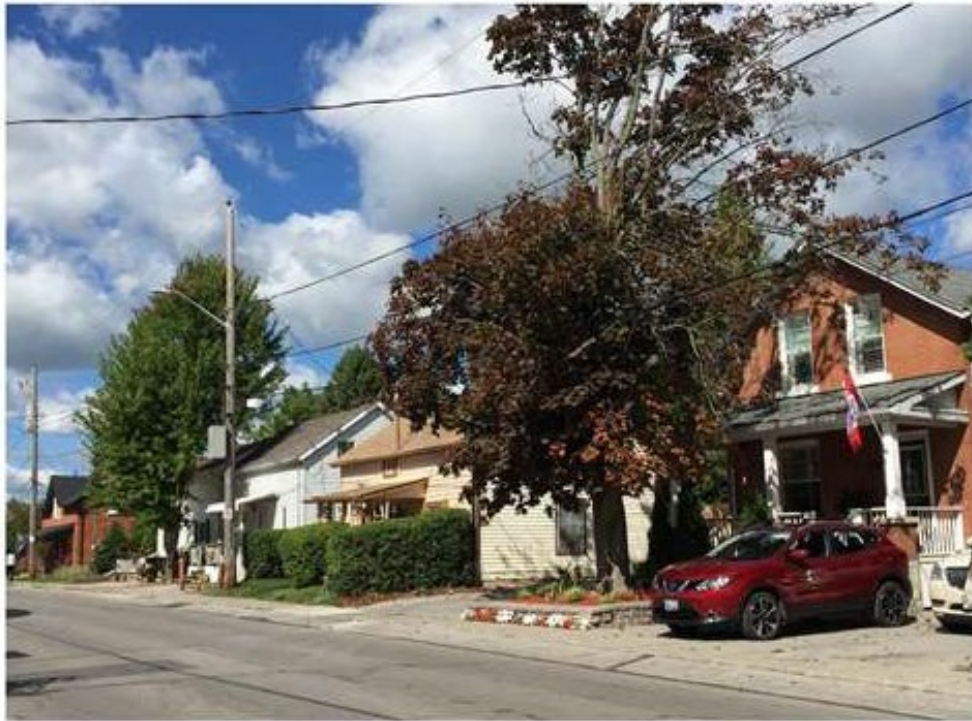
86-108 Albert St. (north side streetscape)
