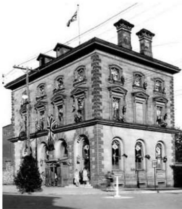
Cobourg Post Office on July 1, 1927. (National Archives.) The original Cobourg Post Office Building was built sometime before 1856 on the southeast corner of Division and King Street, only a little over a block from 93 Albert. In that year Ebenezer Perry sold it to the Bank of Montreal; in 1881 it was conveyed to W. D. Burn who sold it to the Crown in December, 1882. However, it housed the Post Office from 1856 until 1960, when it was demolished and replaced by a new building at Queen and Charles.
