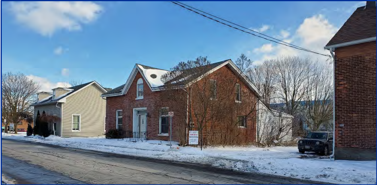
Figure 6: View southeast of the east elevation
