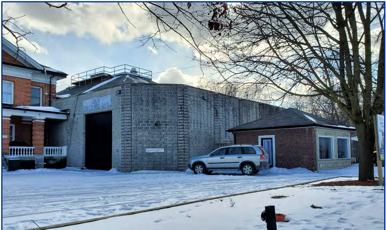
Figure 14: View south of former Cobourg Jail entrance
