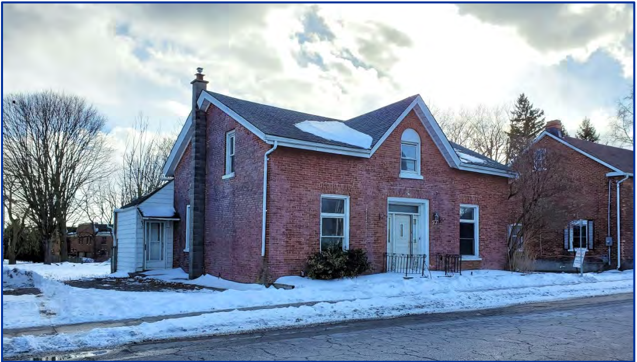
Figure 5: View southwest of the front façade
