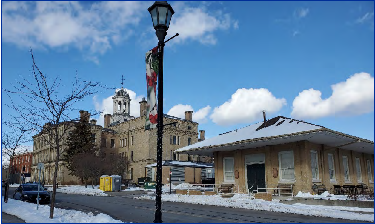
Figure 15: View north of Victoria Hall
