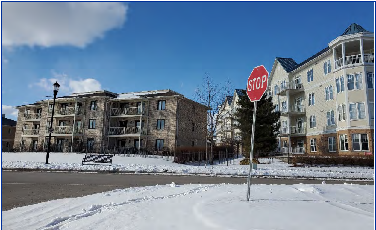
Figure 18: View north of Third Street apartment buildings
