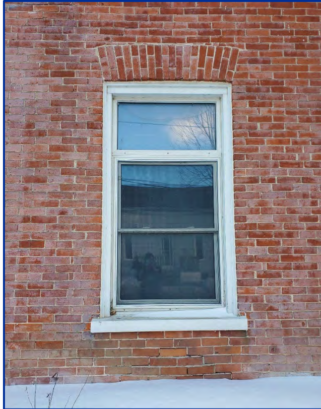
Figure 8: View south of the front window
