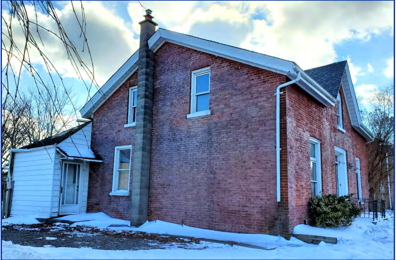
Figure 4: View southwest of the west elevation
