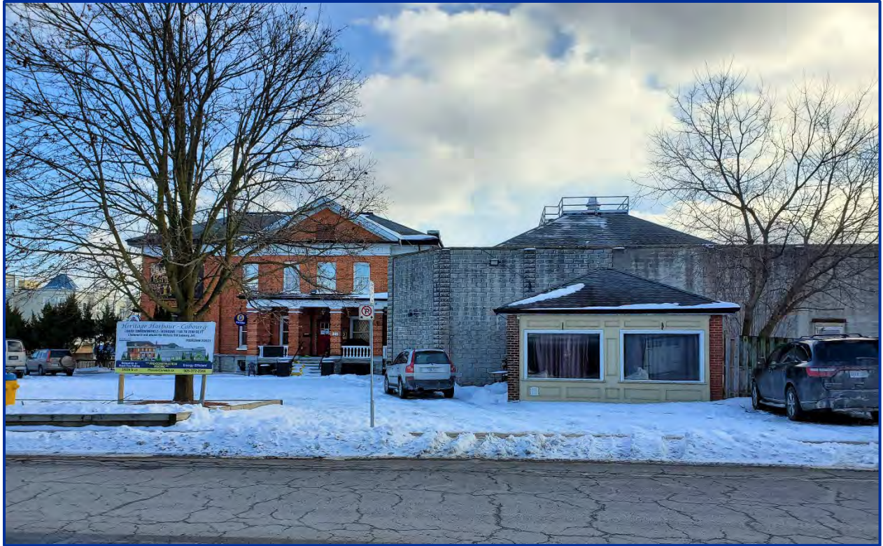
Figure 13: View south of former Cobourg Jail
