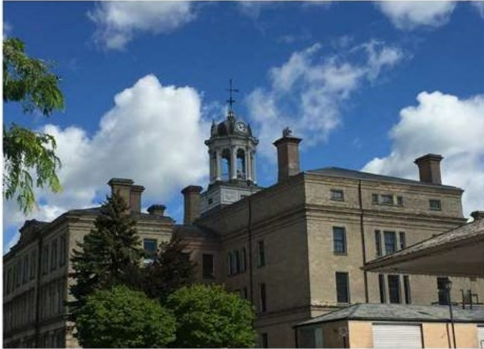
Victoria Hall, south elevation, from Third and Albert Sts.
