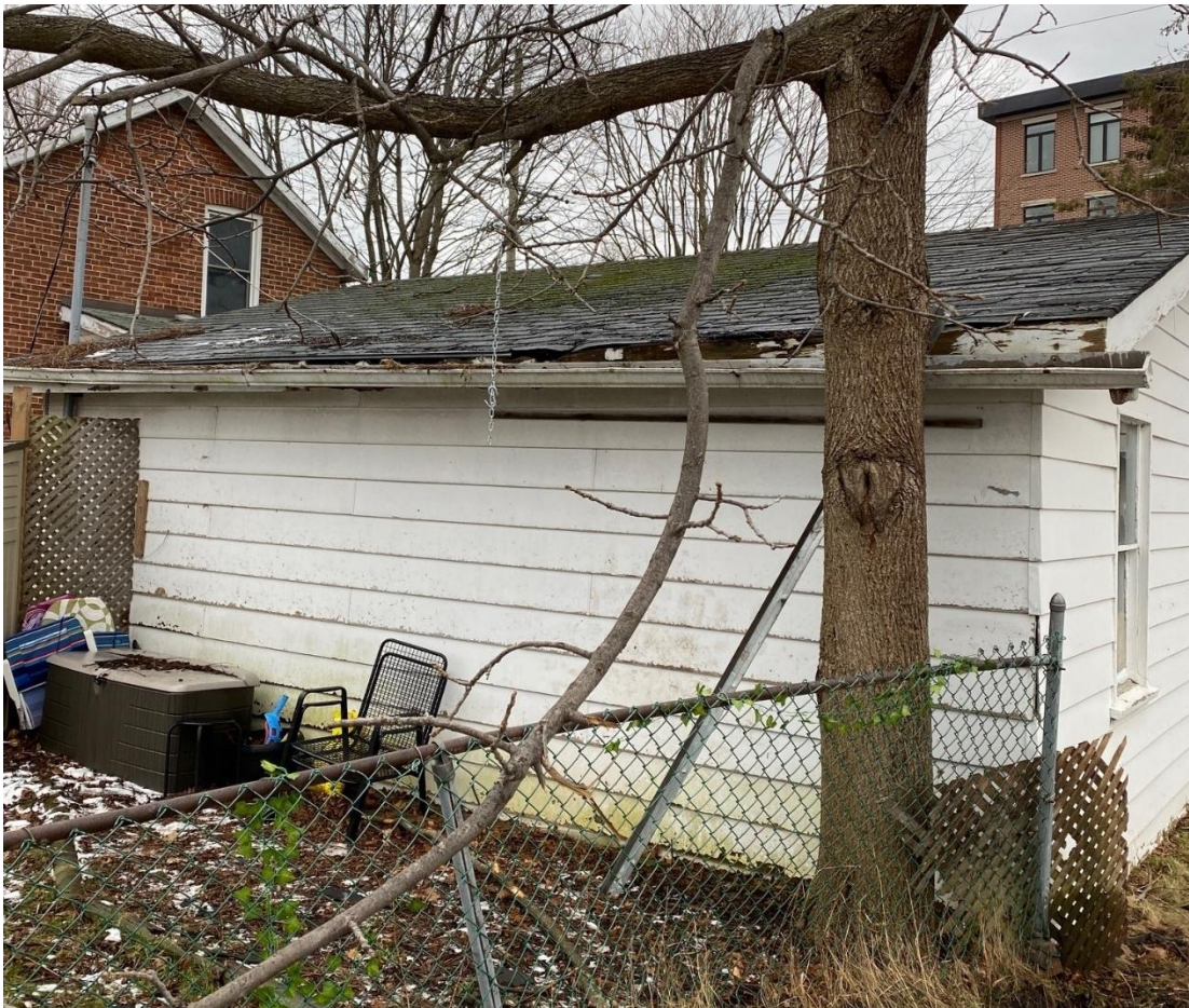
Figure 5: 169 Hibernia St. garage – notice roof and siding condition
