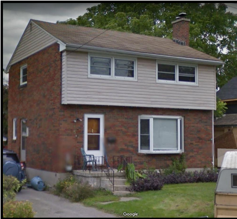
Figure 4: 135 Bagot existing front. Image courtesy: Google
