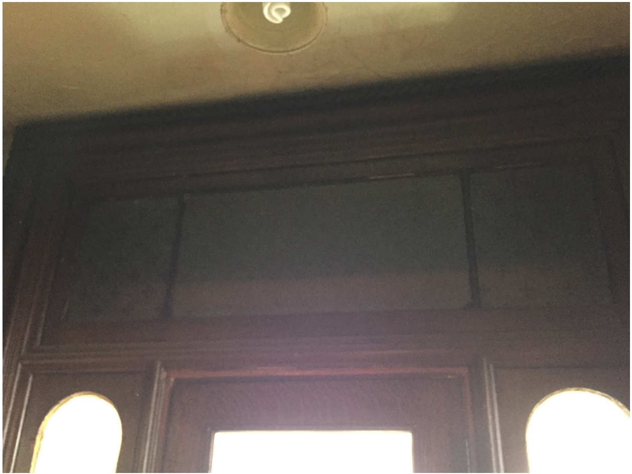
Covered-over front door transom from the inside.
