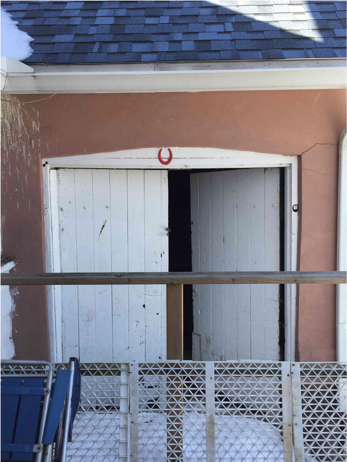
Entrance to drive shed, south elevation
