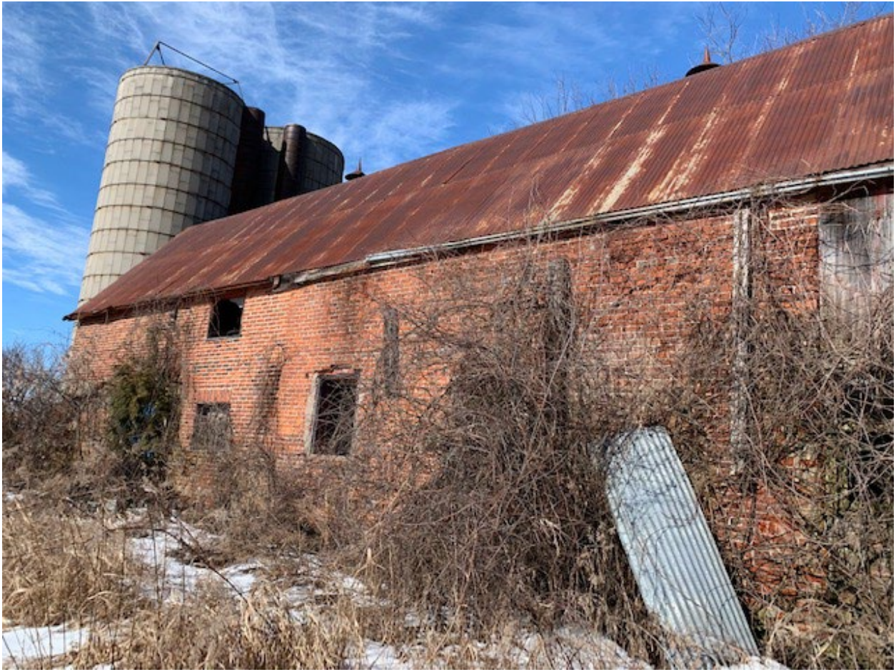
South elevation. Note west end addition
