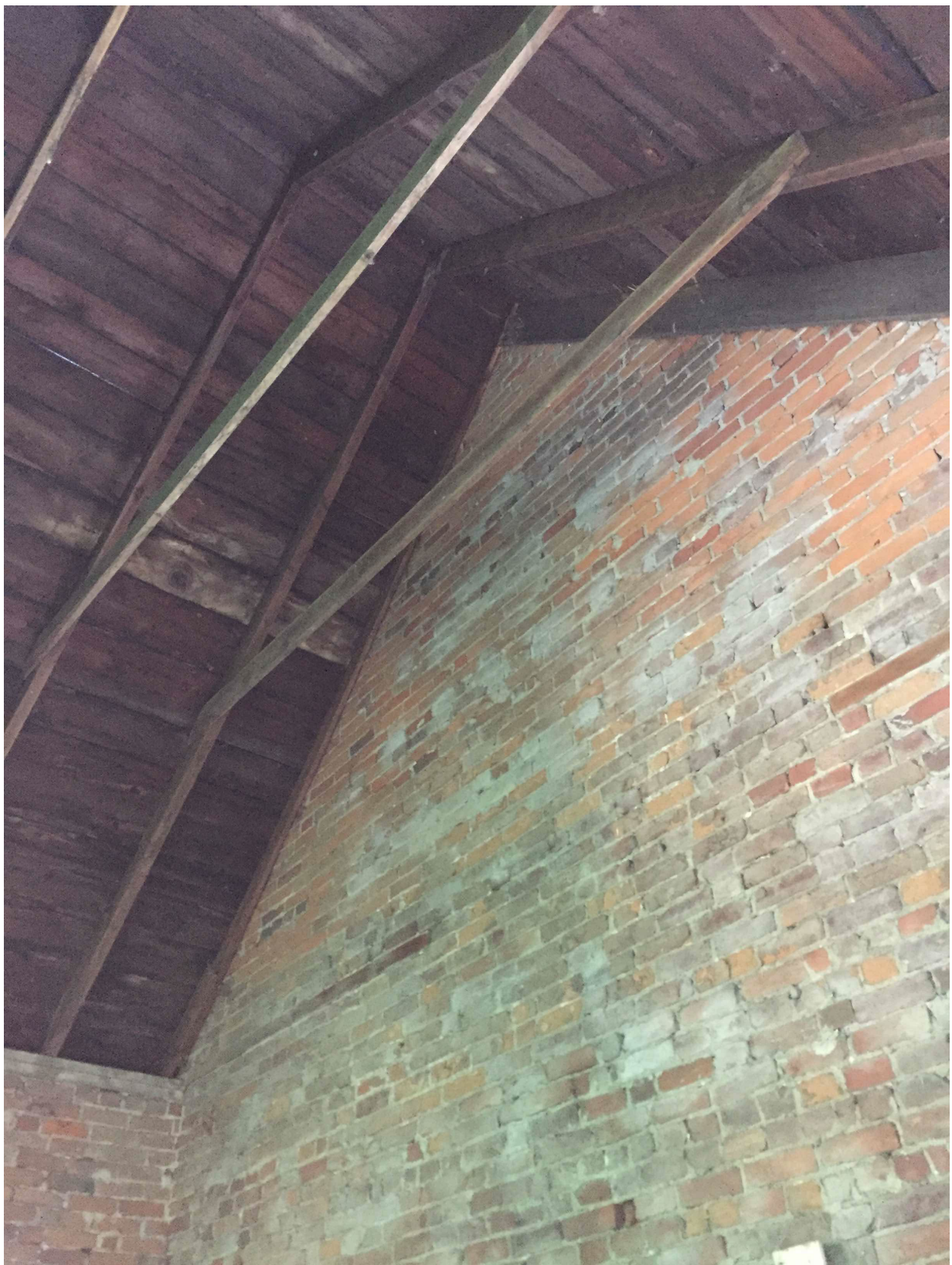
East wall of drive shed from inside
