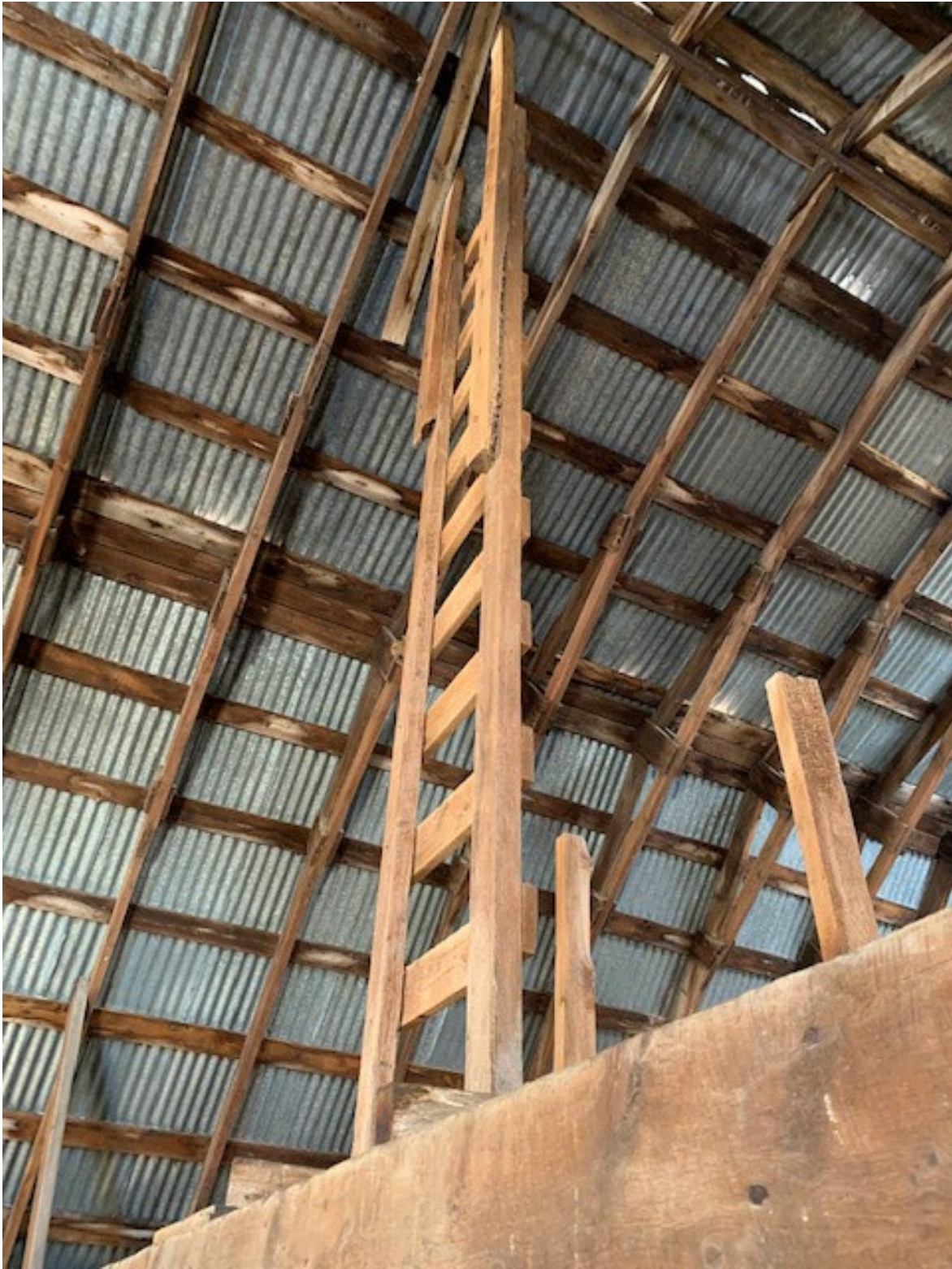
Access ladder in mow
