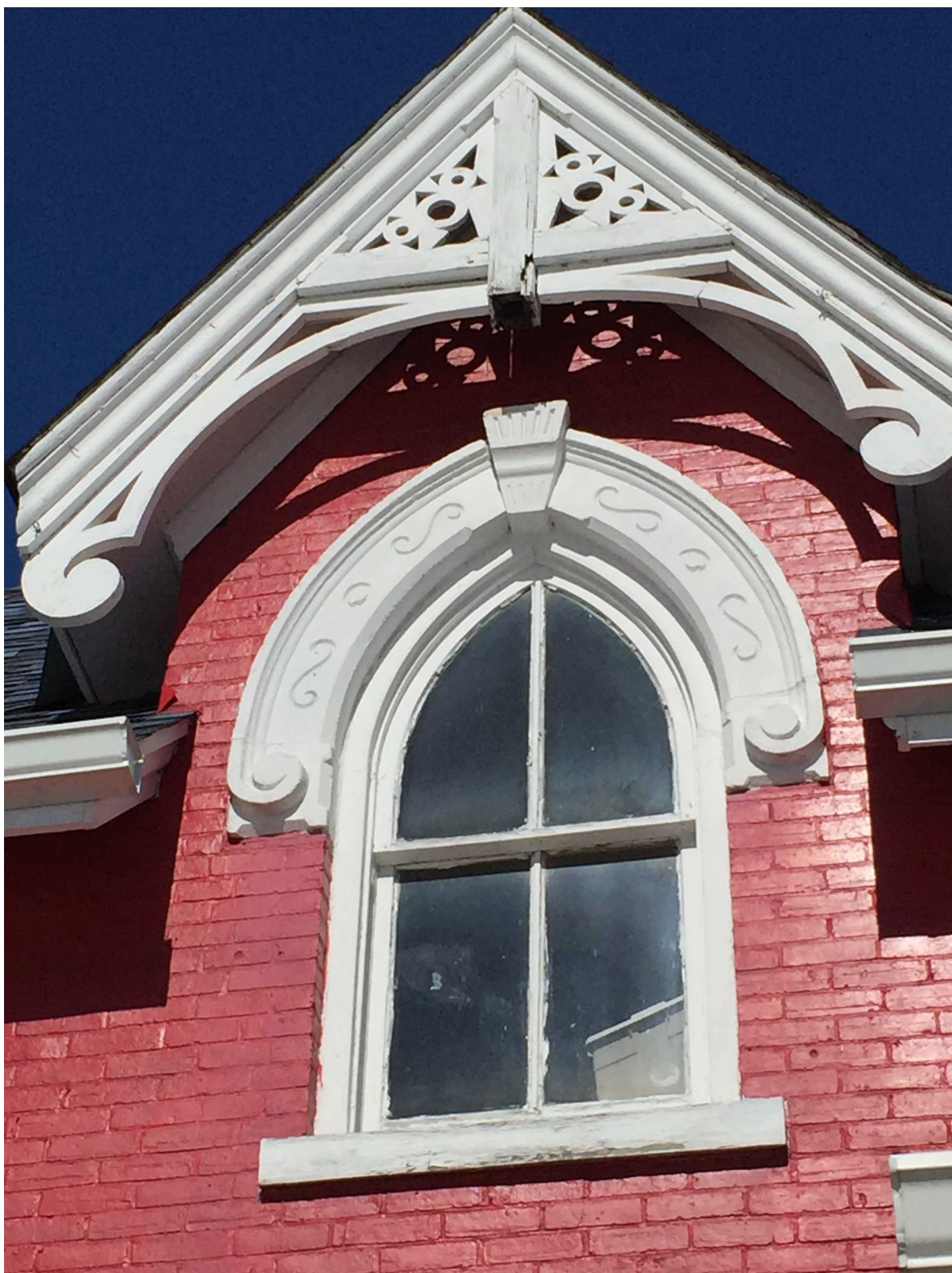
Second-floor dormer with two-over-two lancet window, hood mould, decorative vergeboard, and trusses.
