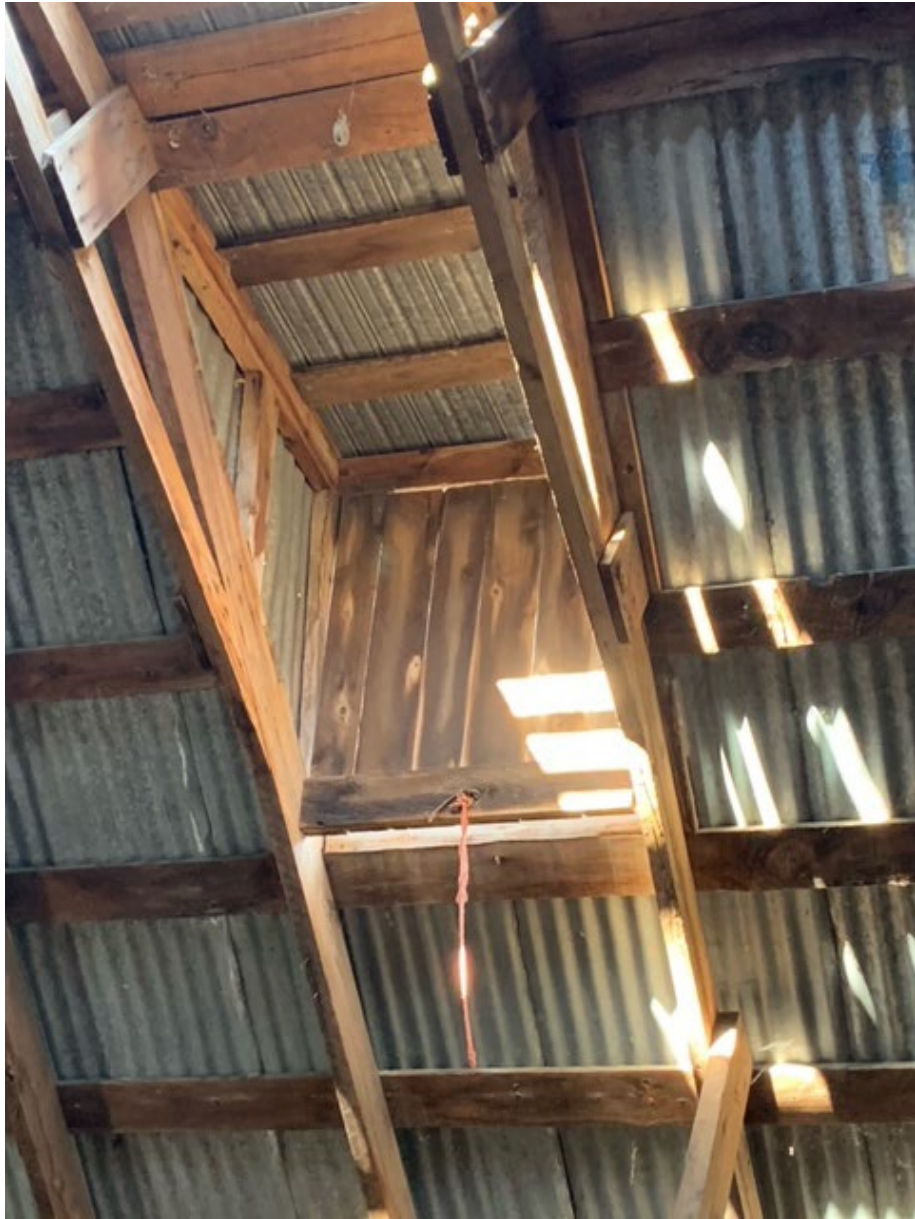
Roof hatch in north elevation
