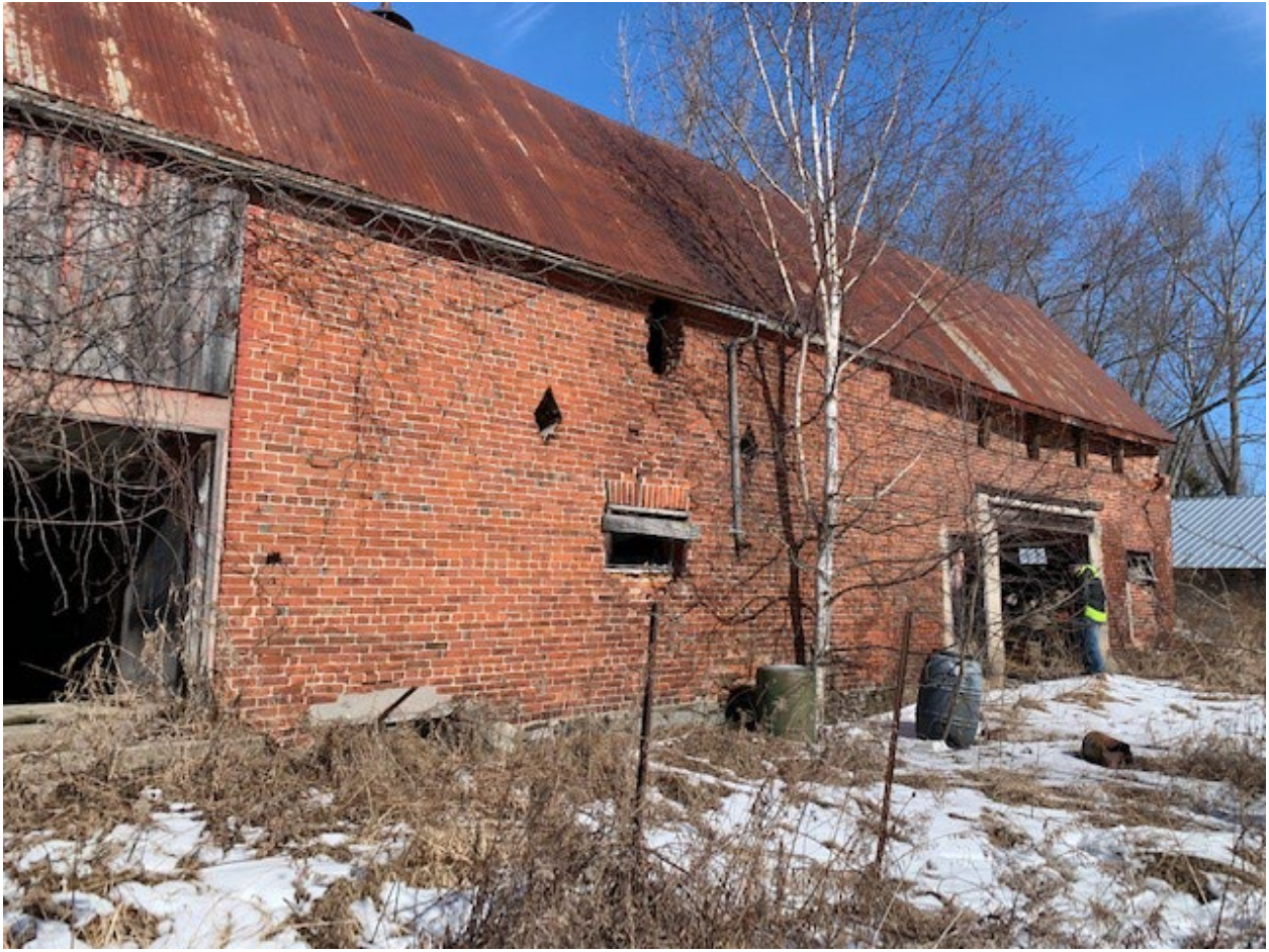
South elevation. Cart doors on left, east end addition on right
