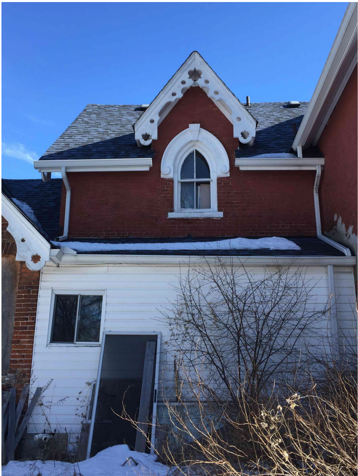
Note different decorative vergeboard pattern on back of house, rear wing, and drive shed
