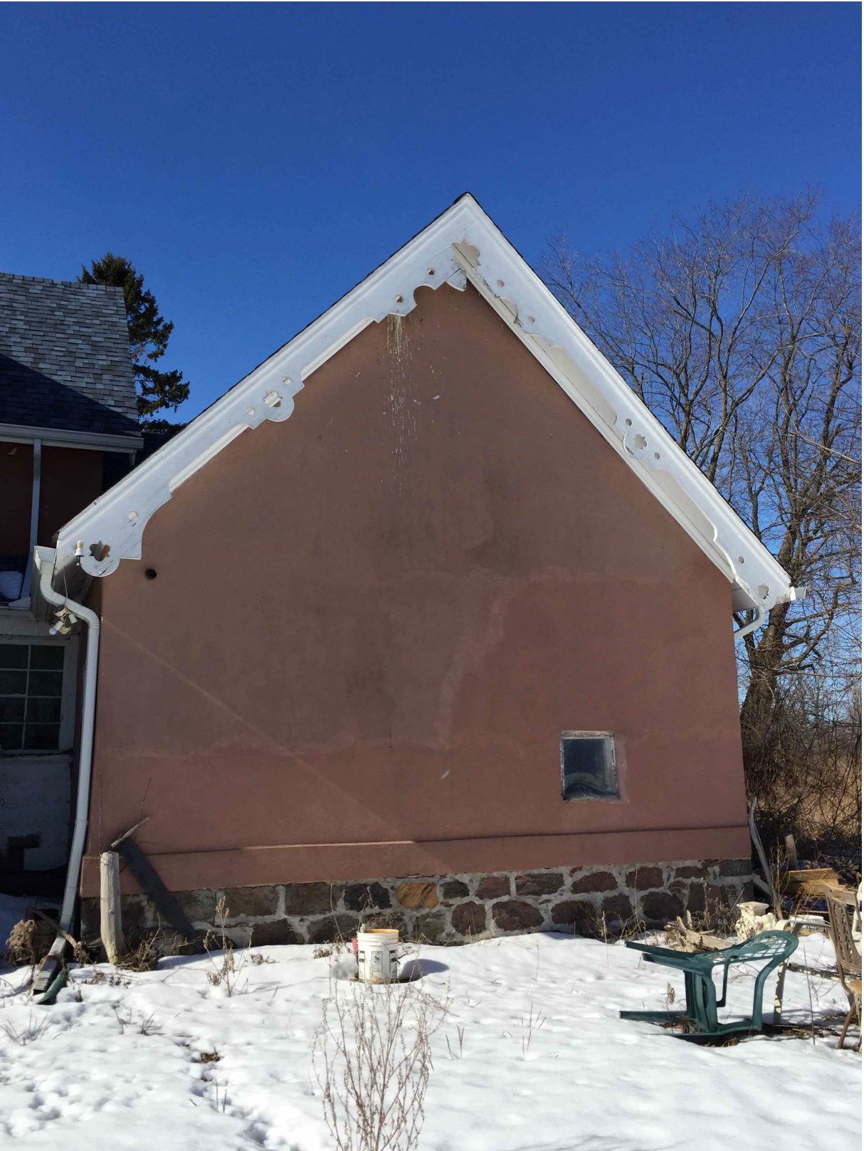
Drive shed, east elevation; stuccoed brick; fieldstone foundation
