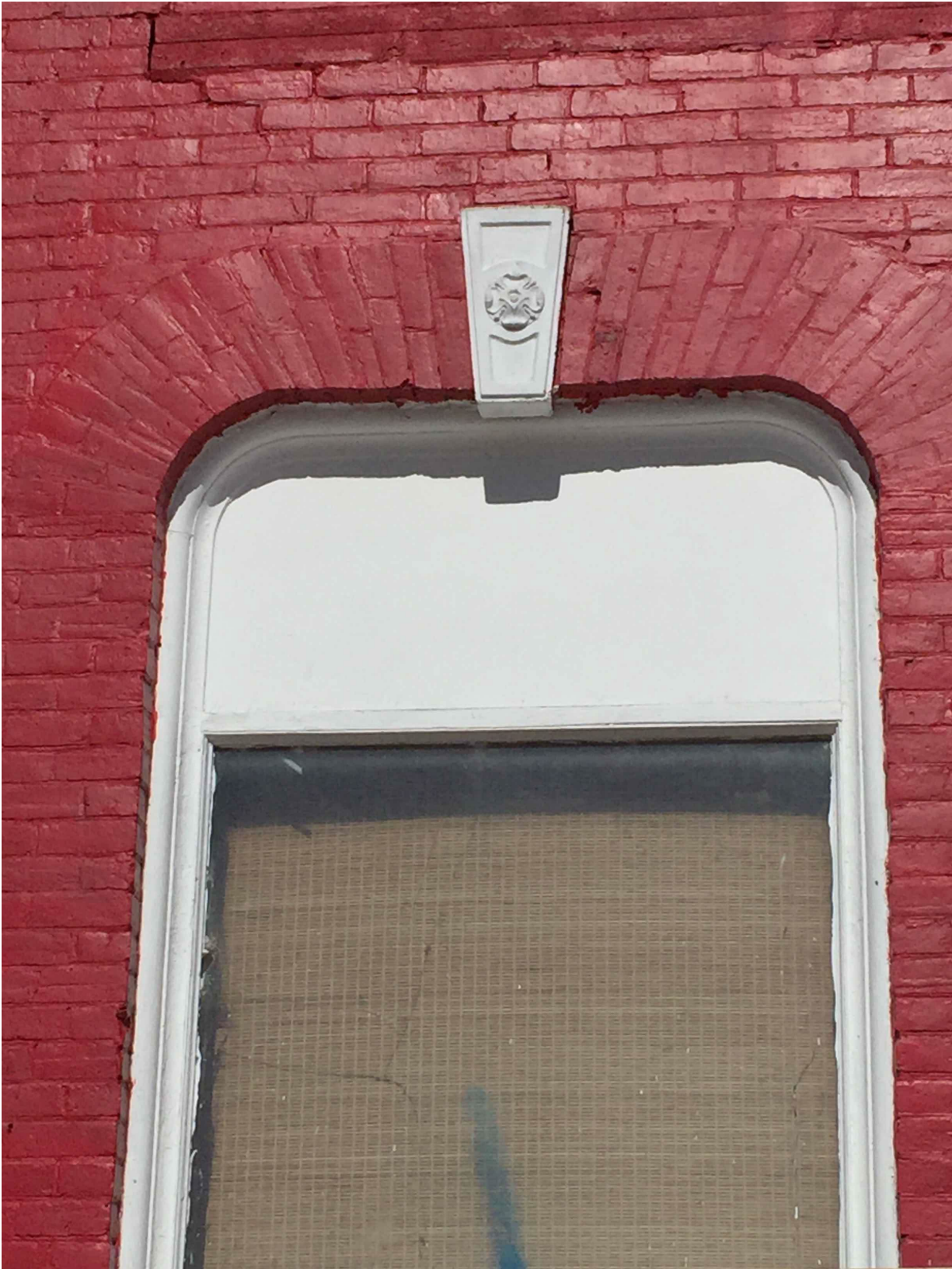
Detail of flattened-arch keystone design and rounded window
