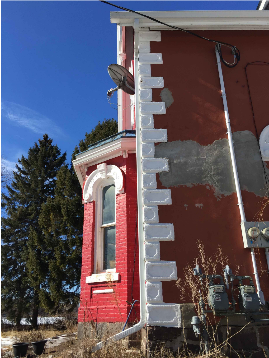
Quoining and the ground-floor bay window, south and east elevations
