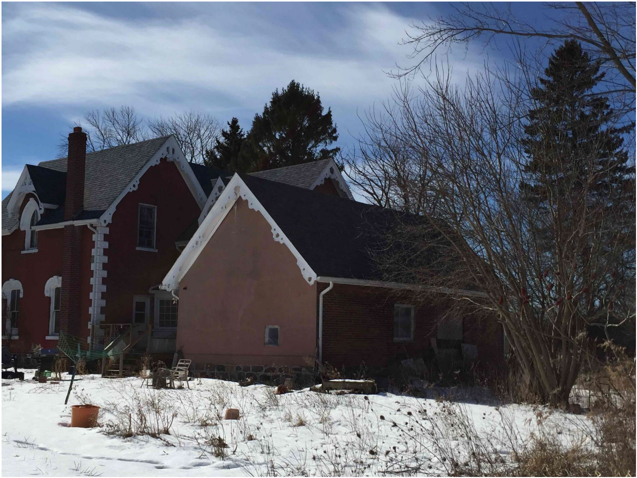
North and east elevation
