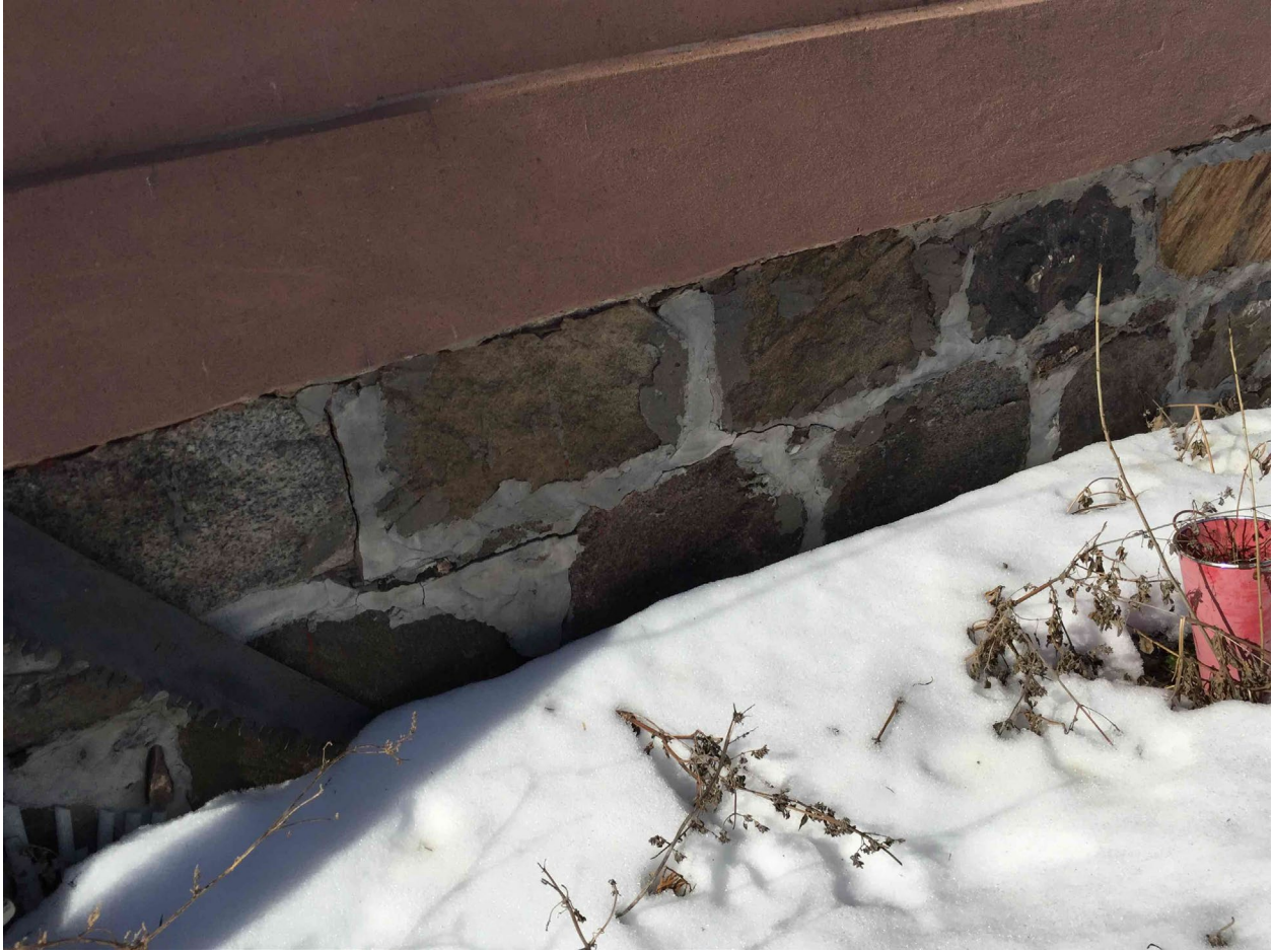
Drive shed, fieldstone foundation
