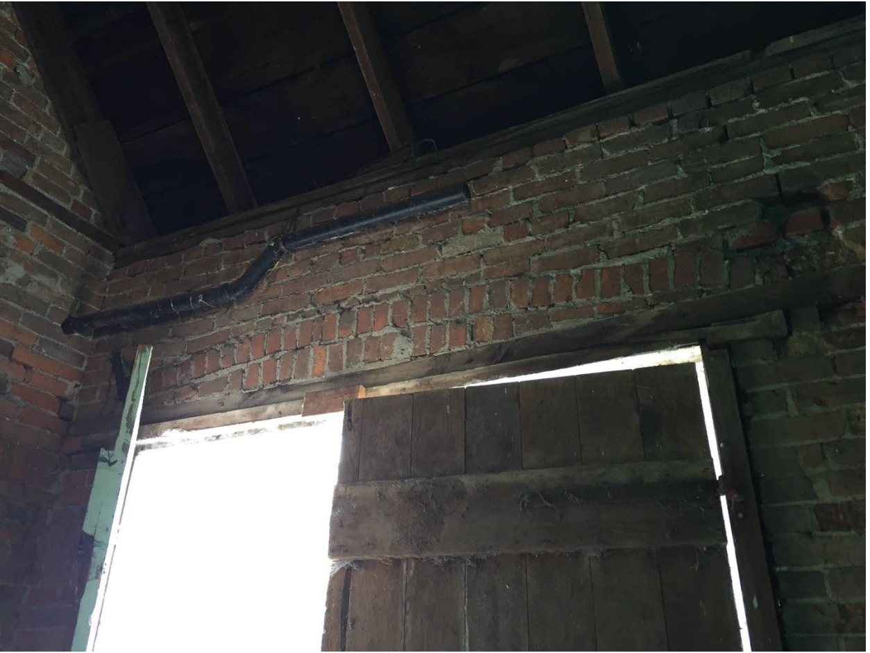
South doors of drive shed from inside
