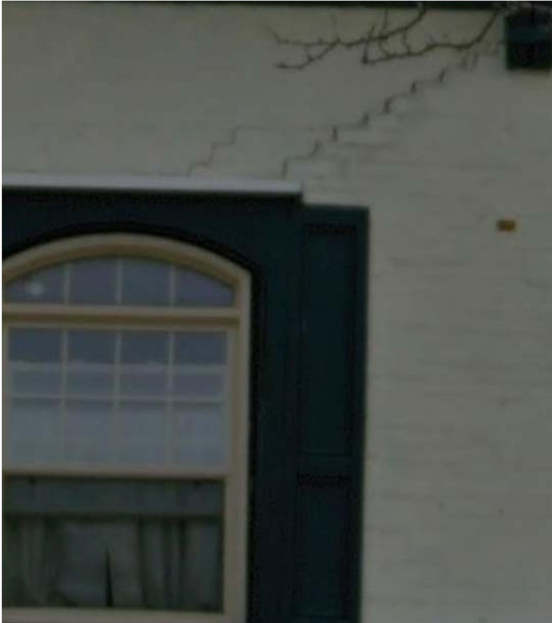
Figure 7: 264 Division St. Masonry crack to be repaired.
