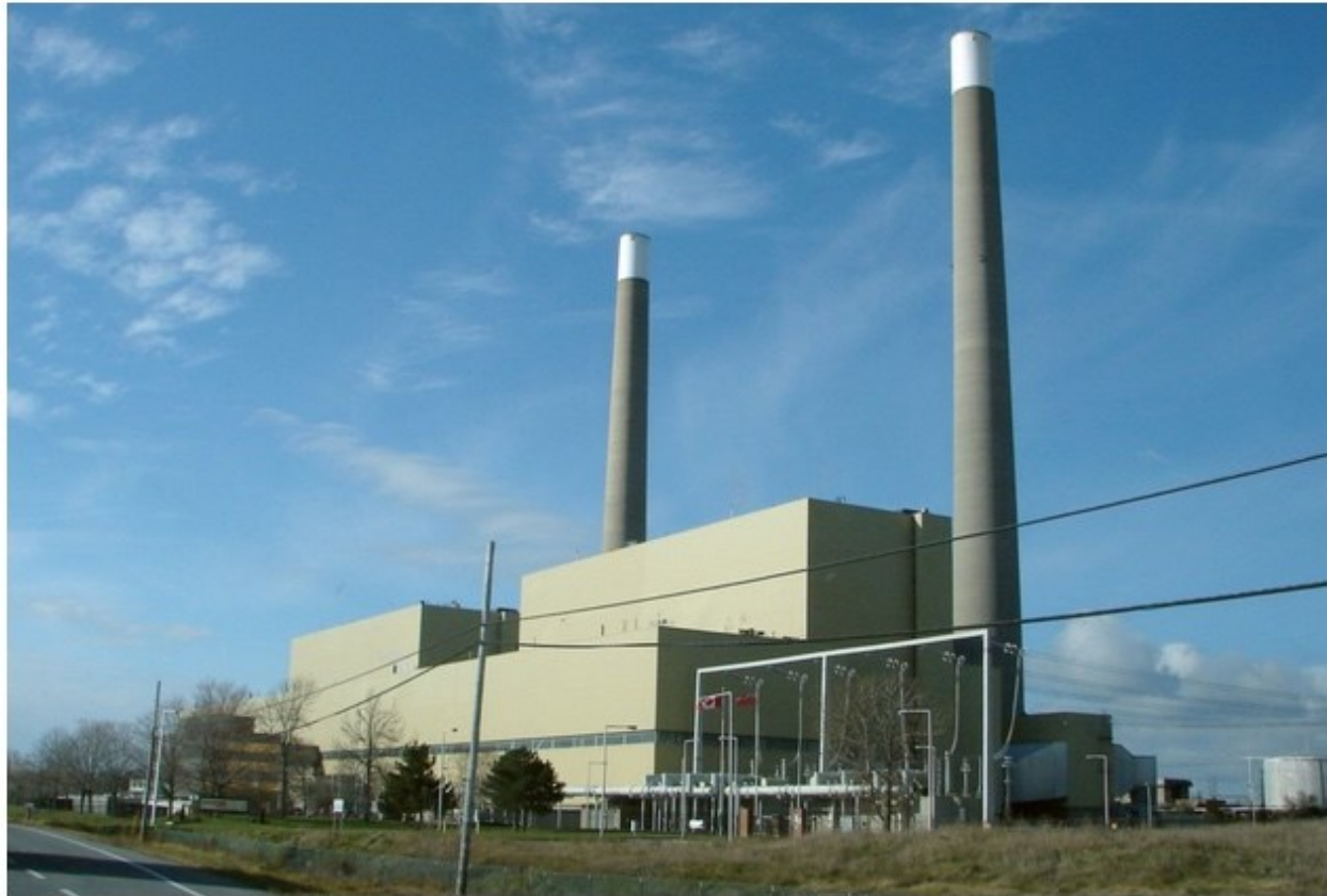
Lennox Power Station near Bath, Ontario, Canada. November 2010.
