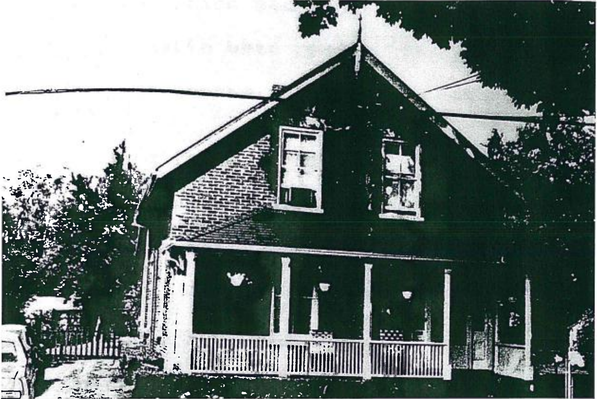
13. 176 Bagot Street. (1985 LACAC Inventory of Cobourg's Century Buildings)
