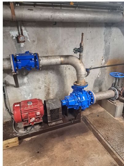
Return Activated Sludge Pump
