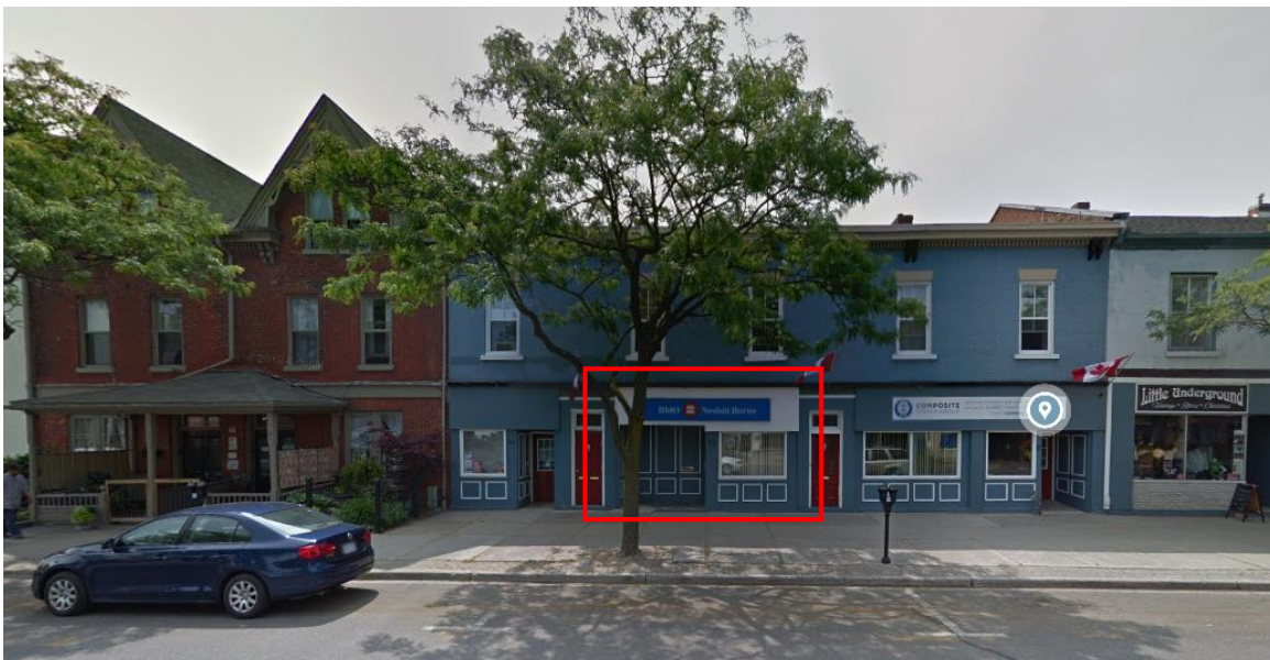
Below: The subject property is shown outlined in red in the context of the streetscape along the south side of King Street.
