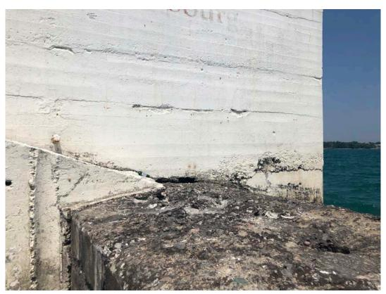
21. Lighthouse, south wall, lighthouse resting on existing concrete breakwater (BA)
