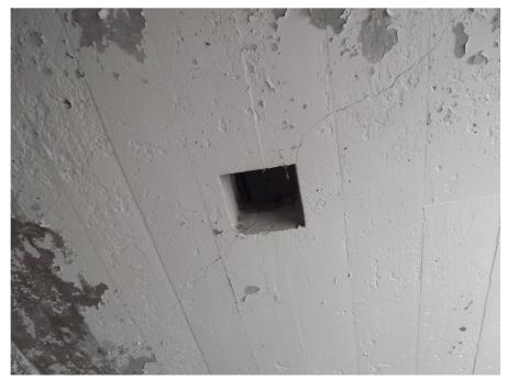
Formed hole in ceiling and ceiling crack
