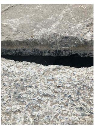
10. East Pier, typical cracking. (BA)
