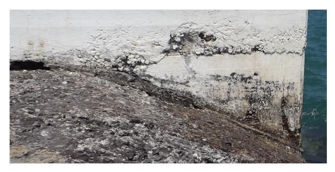
Evidence of levelling base overpour of concrete on existing breakwater
