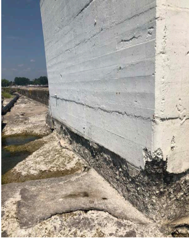
19. Lighthouse, west elevation showing board treatment and erosion at base of wall. (BA)
