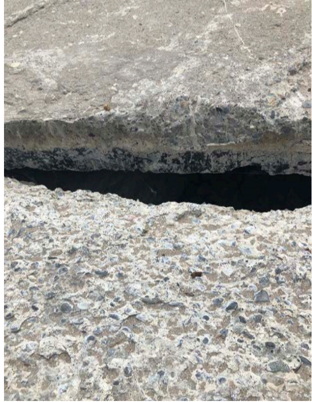
10. East Pier, typical cracking. (BA)
