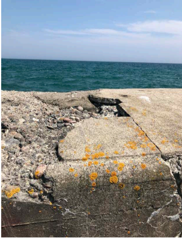
9. East Pier, typical erosion. (BA)
