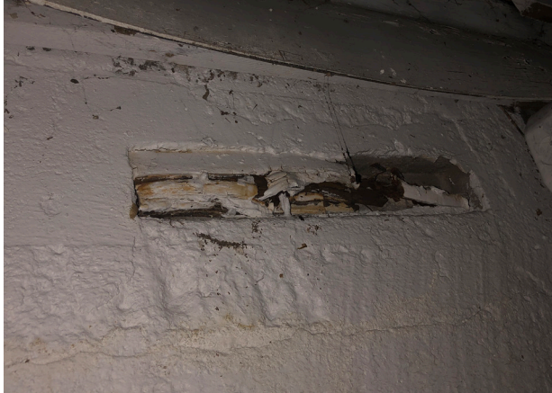
26. Lighthouse, wood blocking in wall. (BA)
