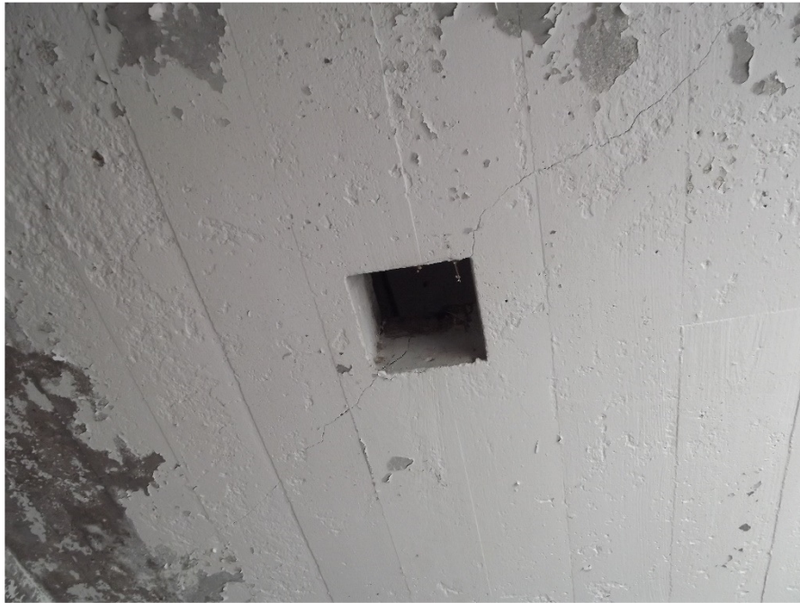
Formed hole in ceiling and ceiling crack
