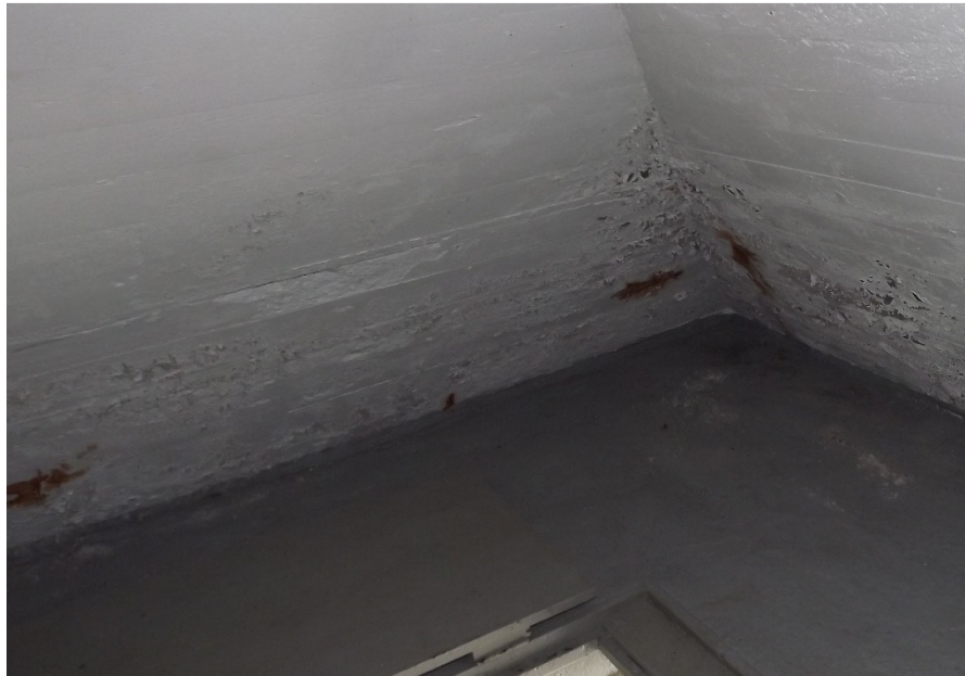
Minor rust stains above the 2 nd level floor
