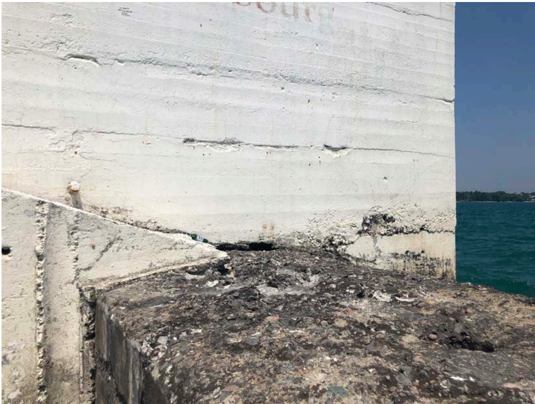
21. Lighthouse, south wall, lighthouse resting on existing concrete breakwater (BA)
