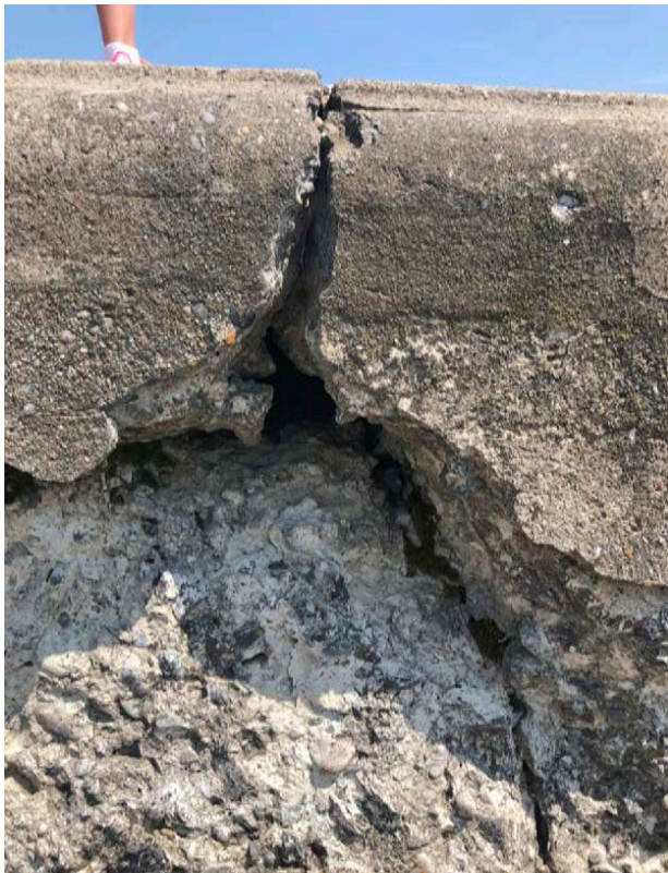
11. East Pier, typical cracking. (BA)
