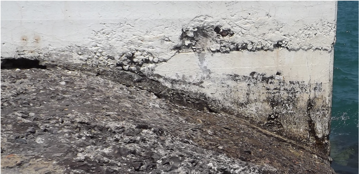
Evidence of levelling base overpour of concrete on existing breakwater
