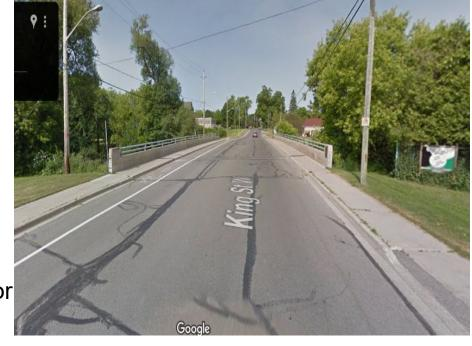
Sanitary, storm and road was constructed in ~ 1960. The bridge over Cobourg Creek requires some minor repairs per 2022 OSIM inspection and a new industrial entrance to WPCP#1 will also be included in the project.
