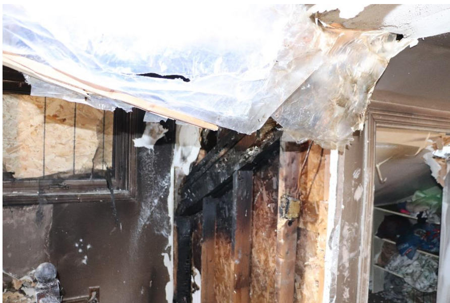
Photograph 10 – Fire damage to knee walls and 2x4 rafters on the western portion
