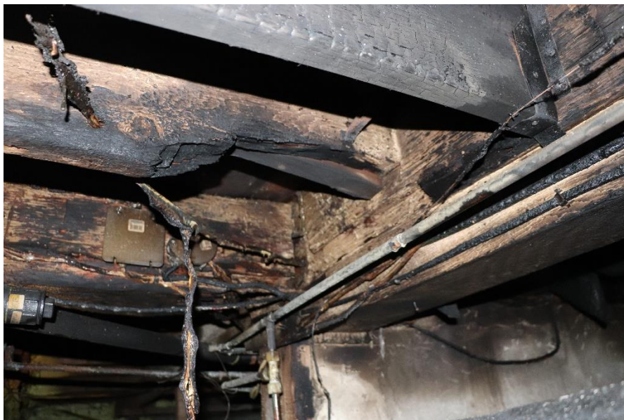
Photograph 8 – Fire damage to adjacent 2x10 floor joists above crawlspace
