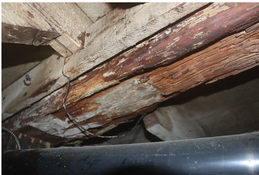
Photograph 9 – Existing, long-term deterioration of timber framing
