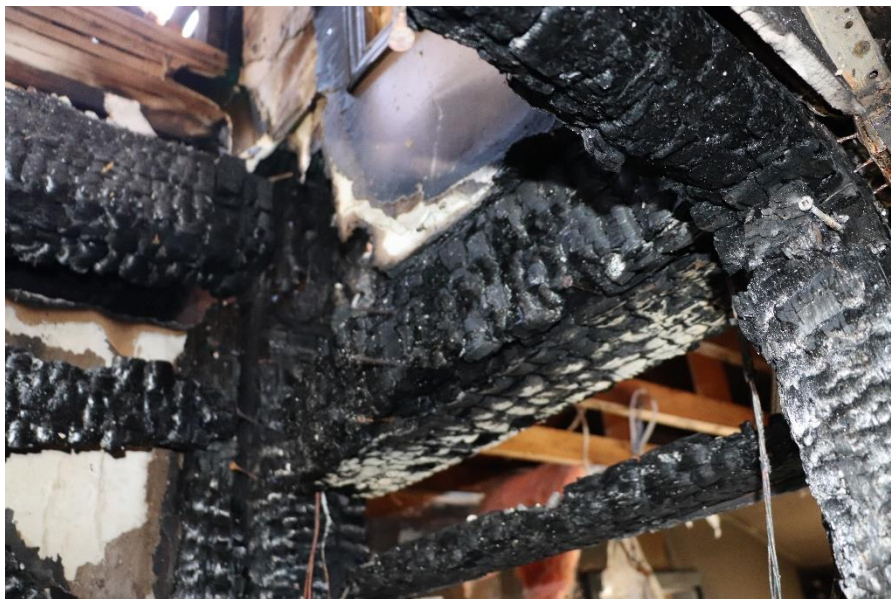
Photograph 5 – Fire damage to timber floor beam and timber columns above
