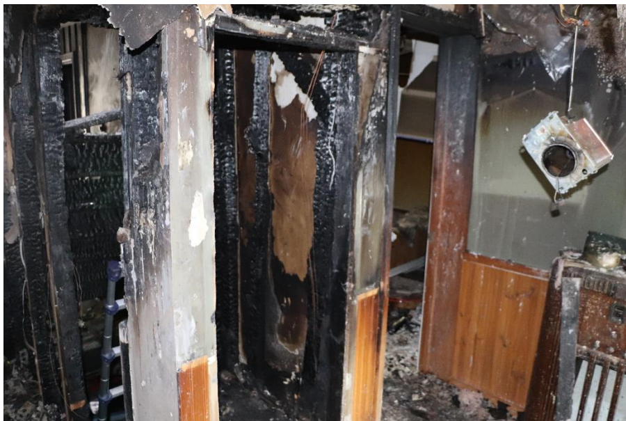
Photograph 3 – Fire damage concentrated around central stairway
