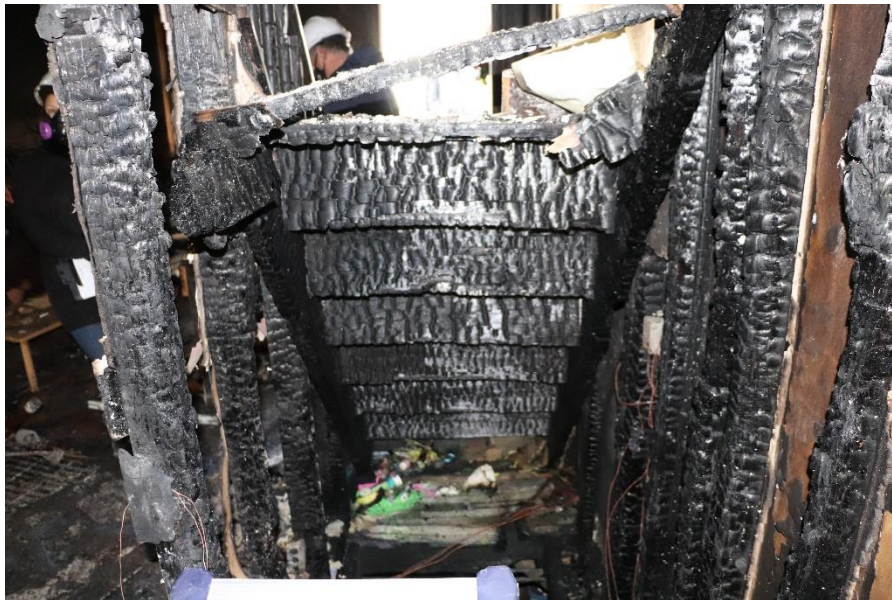
Photograph 4 – Staircase to upper floor partially consumed by fire
