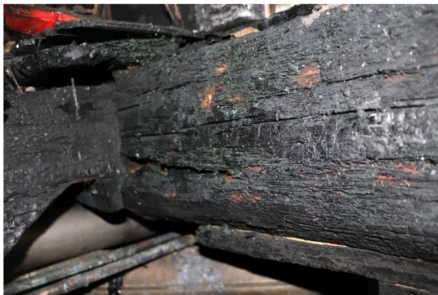
Photograph 6 – Fire damage to central floor beam above crawlspace
