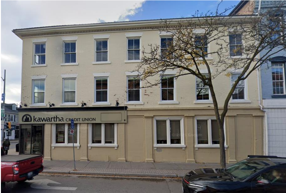
Above: The Subject Property, looking west from Division Street.
