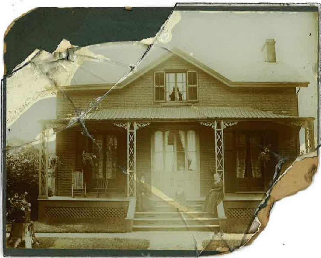
Figure 14. Archival photo showing the principal (north) elevation of the subject property with its front porch with bell-cast roof. (Photo provided by homeowner)
