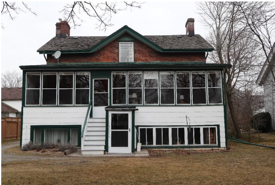
Figure 16. Current photo of rear (south) elevation of 323 King Street West (photo taken by Planning staff during Feb 2024 site visit). The screen door at grade conceals the basement walk-out entrance.
