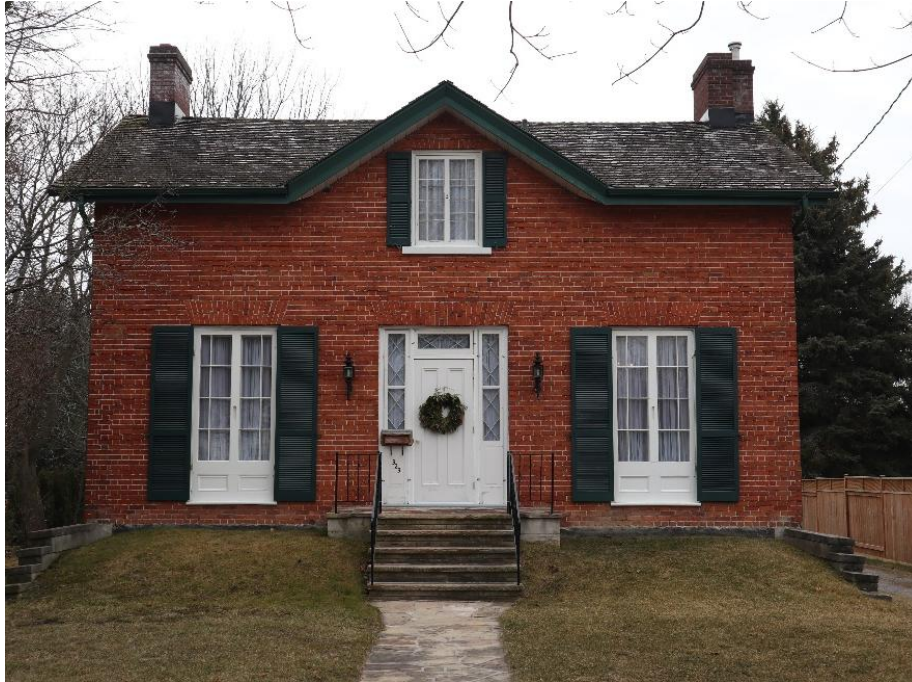
Figure 15. Current photo of principal (north) elevation of 323 King Street West (photo taken by Planning staff during Feb 2024 site visit). Although now absent, the verandah would have contributed to the dwelling's horizontal emphasis. The curved bell-cast roof would have made the wide expanse of roof appear lighter and more graceful 62 .
