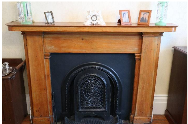
Figure 22. Fireplace in dining room (photo taken by Planning staff during Feb 2024 site visit)
