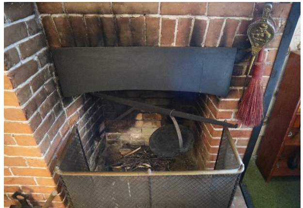
Figure 24. A close-up photo of fireplace crane (photo taken by Planning staff during Feb 2024 site visit)
