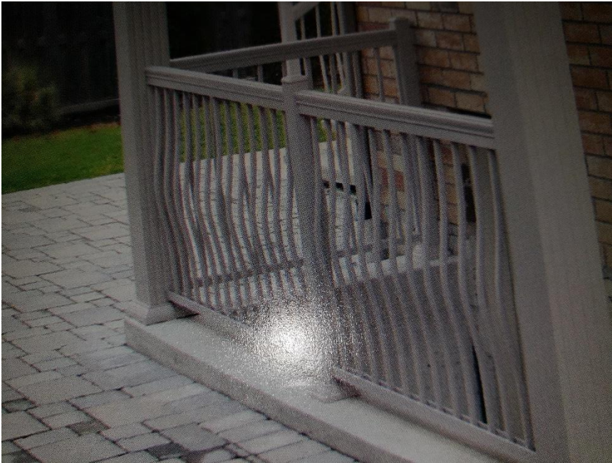
Figure 7: Proposed railing system from AlumaRail – colour to be white (Please see Appendix 1 for the product brochure) – Rail system is on page 3 and is highlighted. This railing must be designed to comply with Building Code requirements for height, spindle separations and safety/stability.
